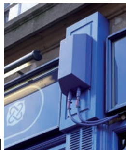
Microcell providing extra capacity in town centre
